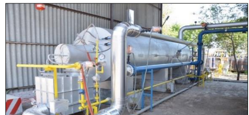
Figure 3: Furnace with Regenerative Burners on either ends
