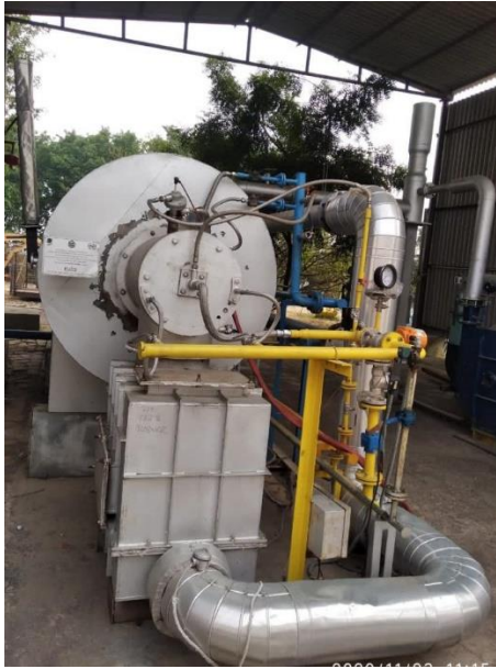
Figure 2 – Regenerative Burner System
